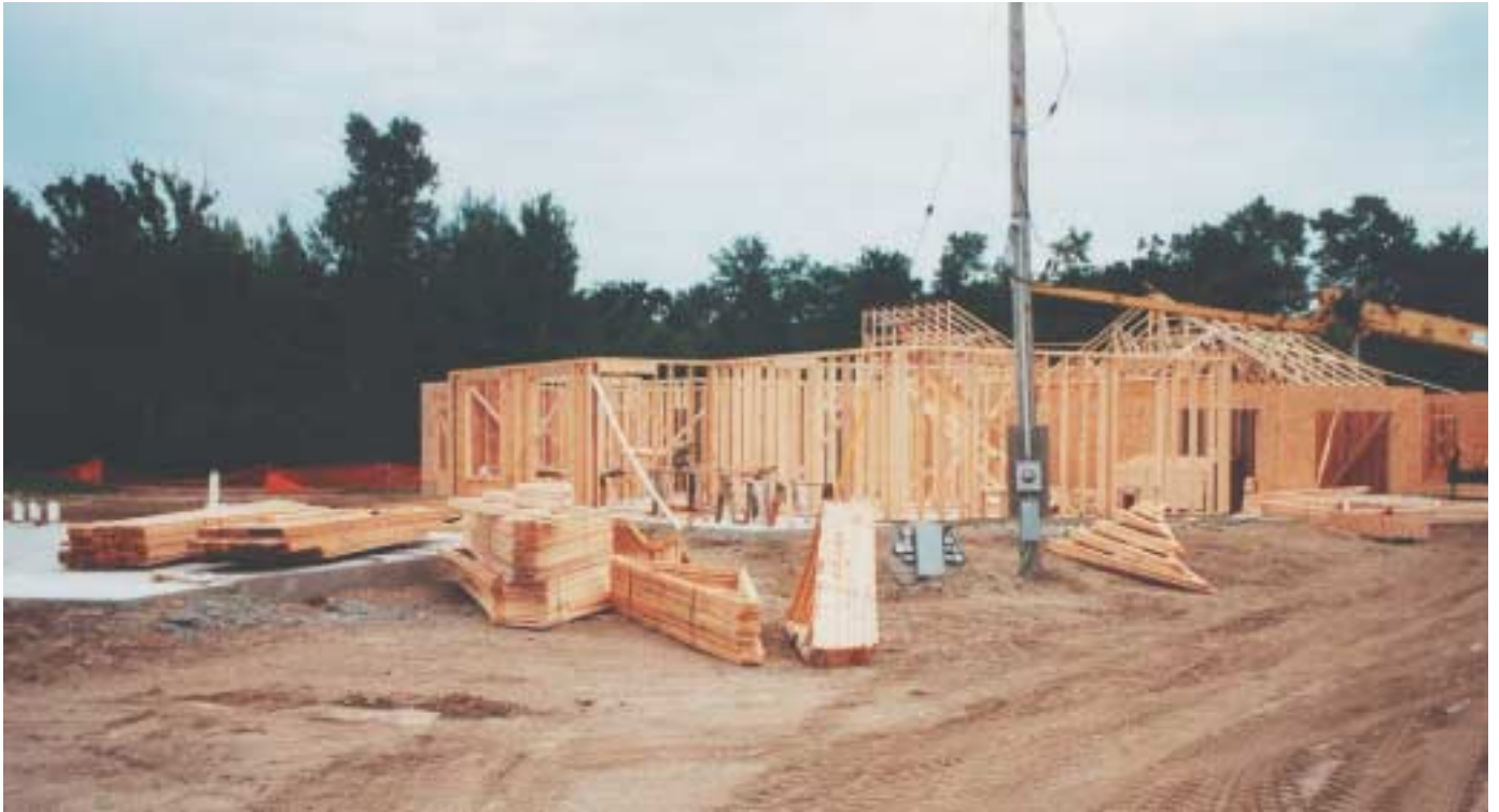
Walls ready to receive trusses on a multi-family project.
