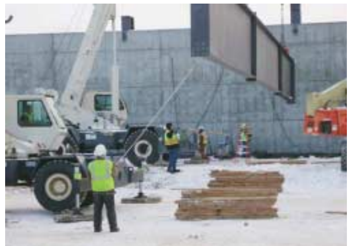
Massive beams being erected at the Urban Plains Center.
