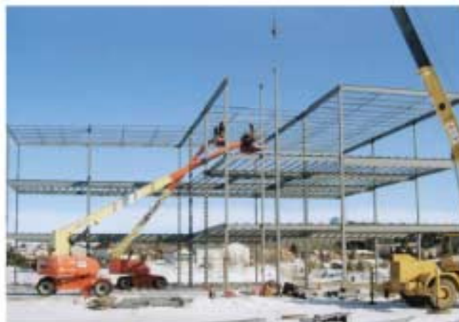
The three-story primary steel structure being erected.
