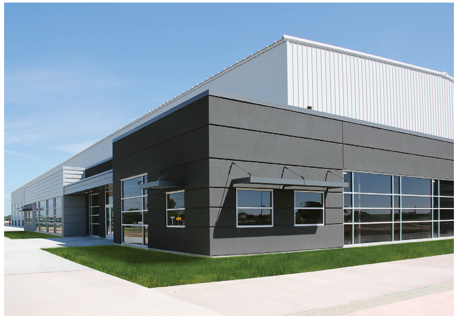
A close-up focusing on a few of the building's features: EIFS (exterior insulation finishing system), sunshades and windows.
